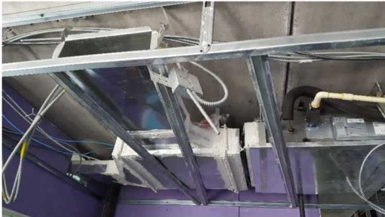
Ducted Ceiling Units
