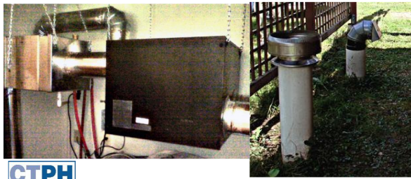
30" thick 18 th century stone walls: night time ventilation cooling (8hr lag time)
