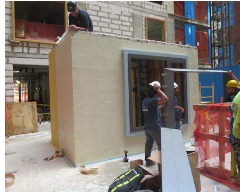
An extensive mock-up could be a full six-sided box with various details reflected.
