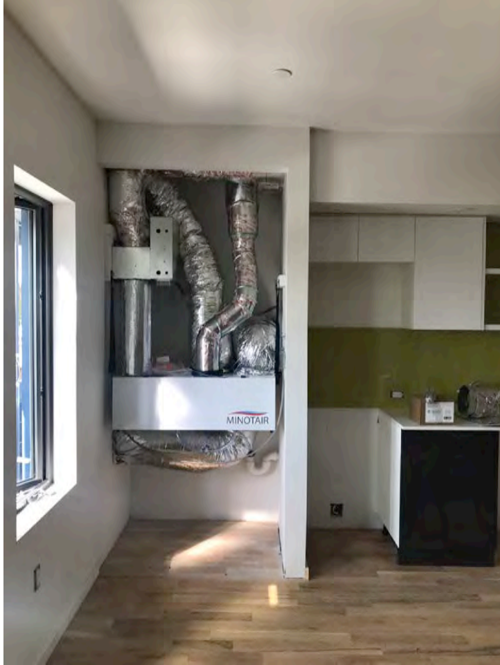
HVAC Closet merged with Kitchen cabinetry
