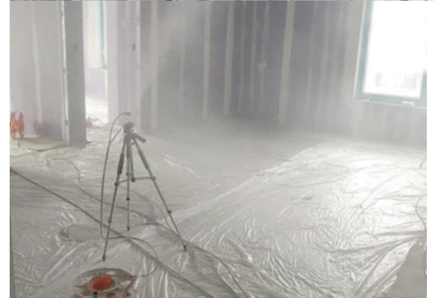
Vaporized Sealant
