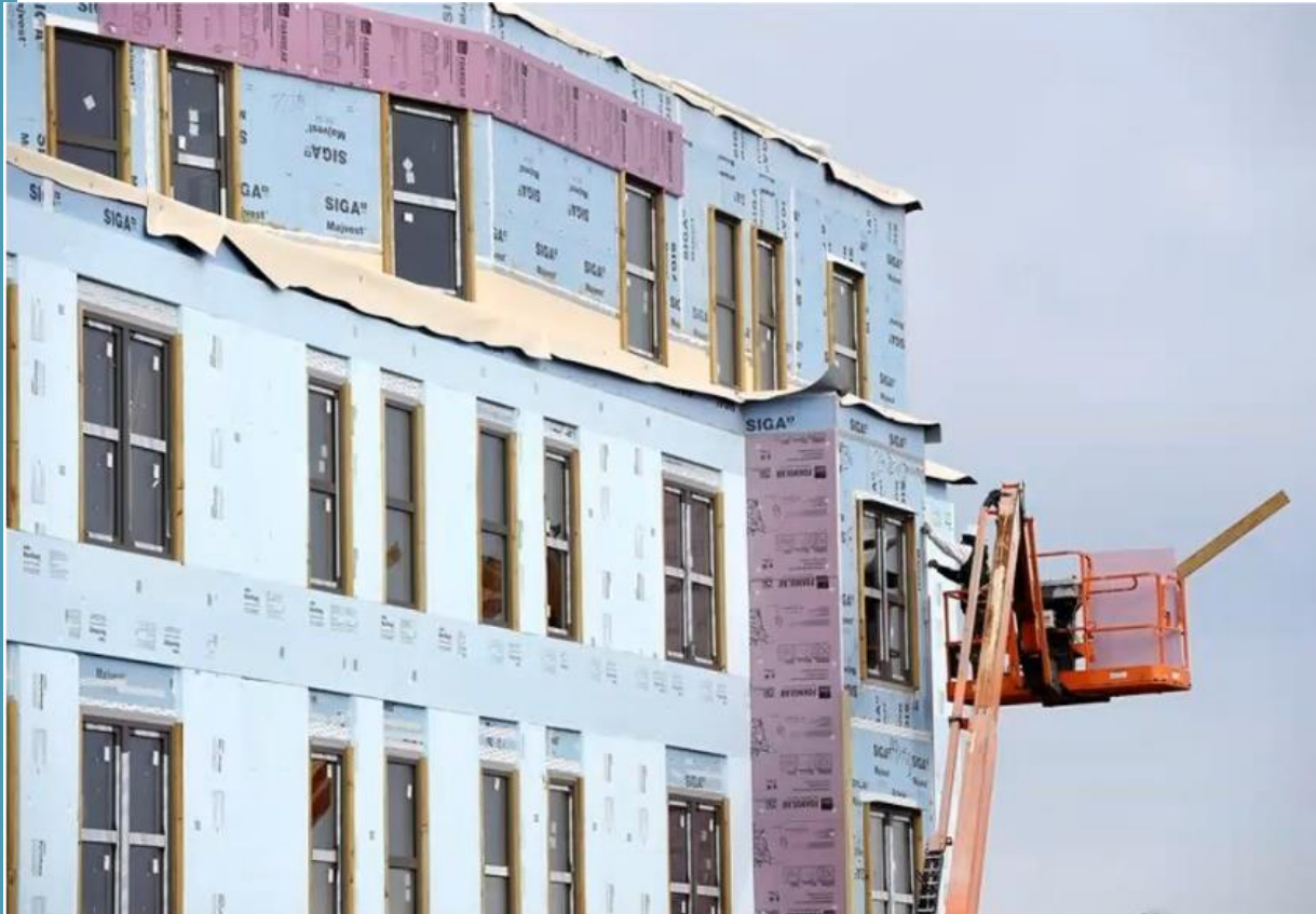
Harbor Village: Dense Foam insulation over Siga Airbarrier system
