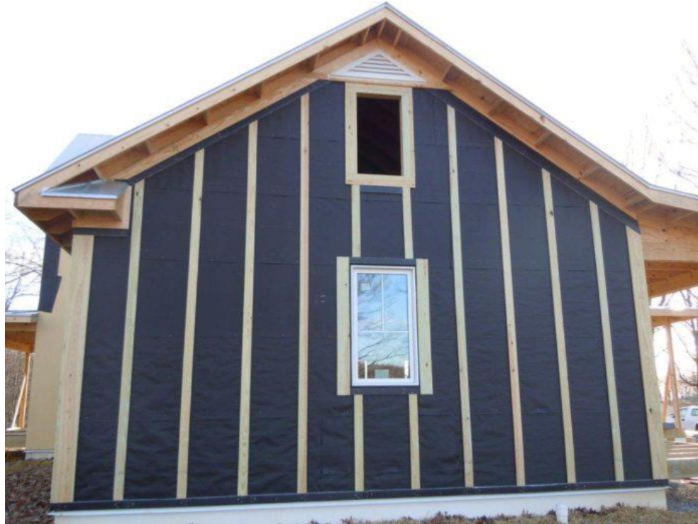
Rainscreen with vertical strapping and coravent at top and bottom of wall
