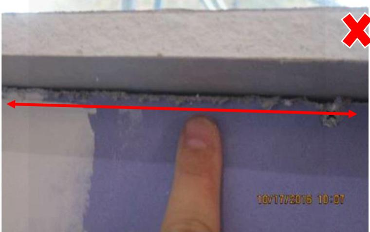
Unsealed gap between bottom of sill & drywall
