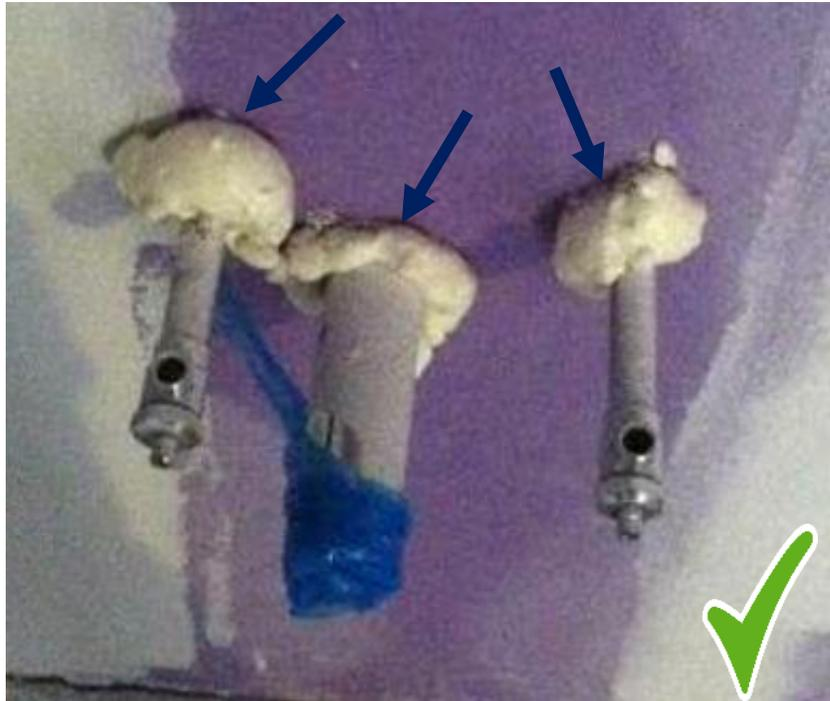
Sealed Kitchen sink penetration with spray foam/caulk
