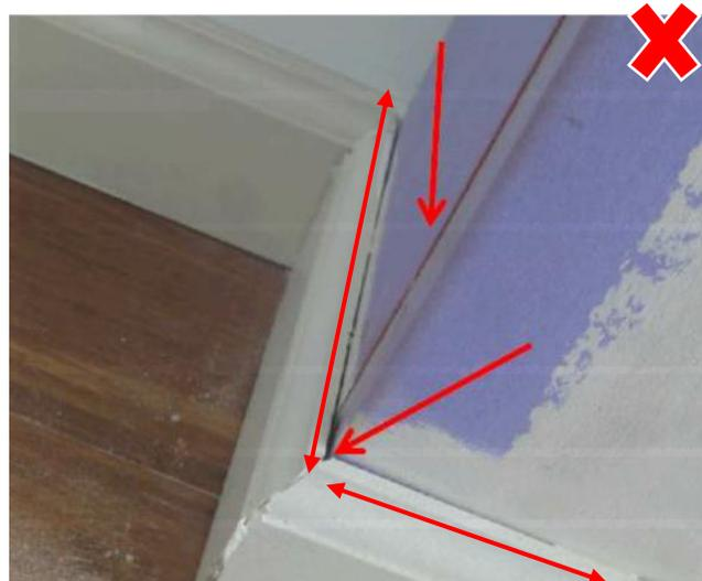
Unsealed gaps between floor and dry wall/base molding
