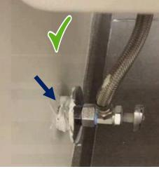
Sealed Toilet penetration with spray foam/caulk
