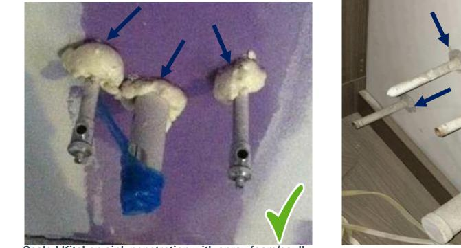
Sealed Kitchen sink penetration with spray foam/caulk
