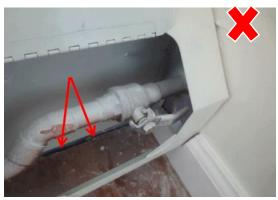
Unsealed gaps between floor and dry wall/base molding
