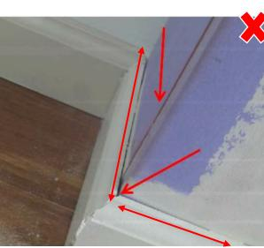
Unsealed gaps between floor and dry wall/base molding
