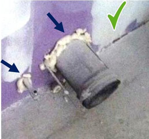
Sealed Toilet penetration with spray foam/caulk
