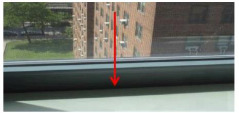
Gap between frame of window & drywall
