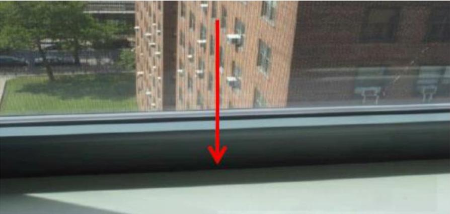
Gap between frame of window & drywall
