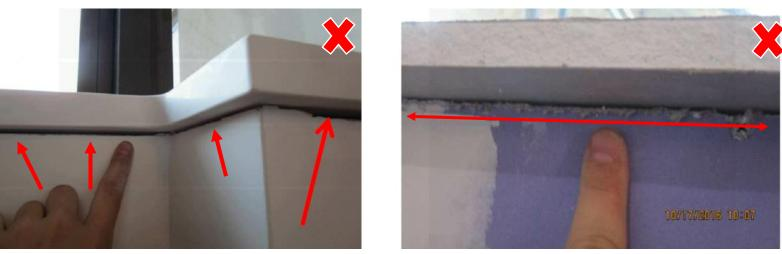
Unsealed gap between bottom of sill & drywall
