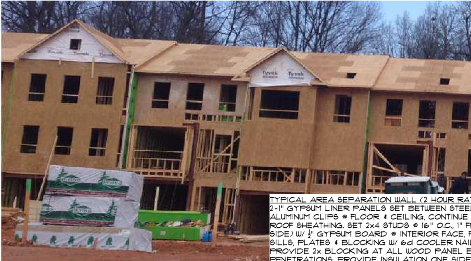
TYPICAL AREA SEPARATION WALL (2 HOUR RATED - UL #U336)
