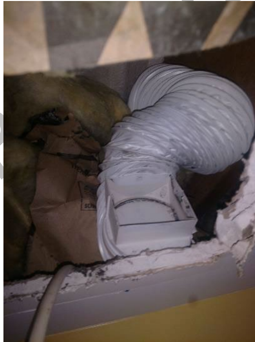
Flex duct poorly installed
