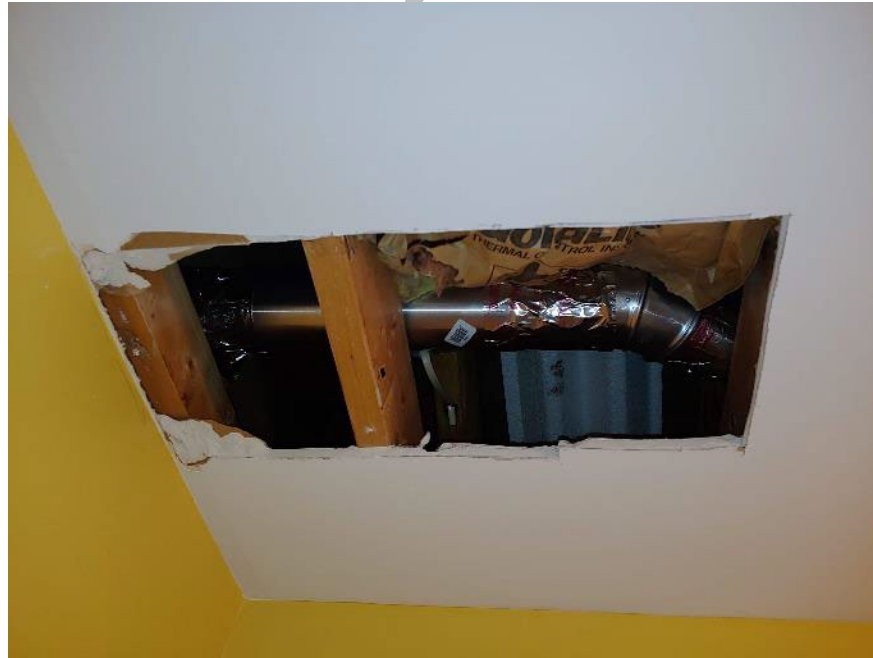
Straight, hard ducted run
