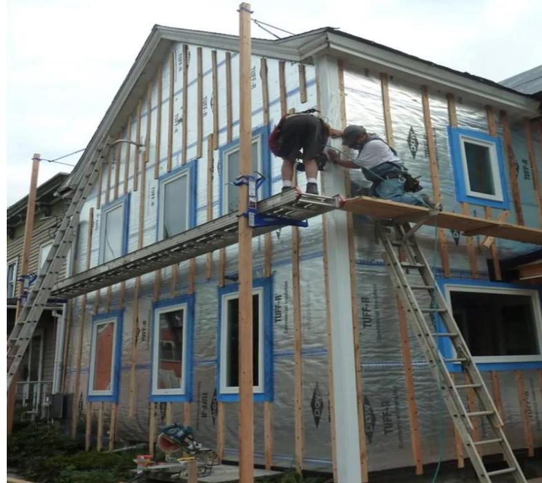
Rainscreen w/ 1x3 strapping provides 3/4" drainage and ventilation gap
